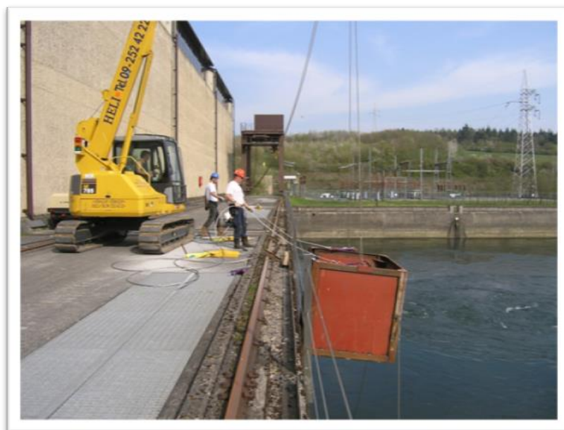
Photo n° 17: Setting of the protective chamber
