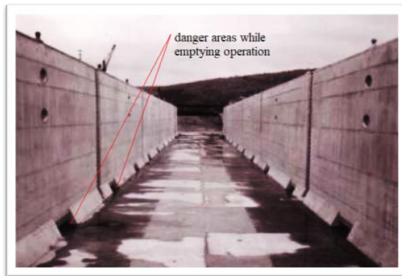
Fig. n° 25: Illustration of delta P risks due to longitudinal culvert
