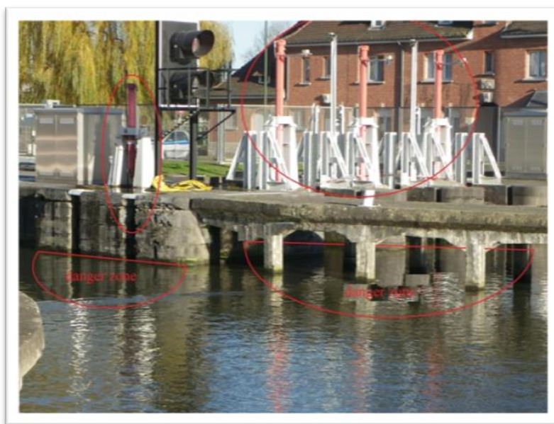
Photo n° 29: Upstream culvert inlet with protection grid (doc. Internet)
