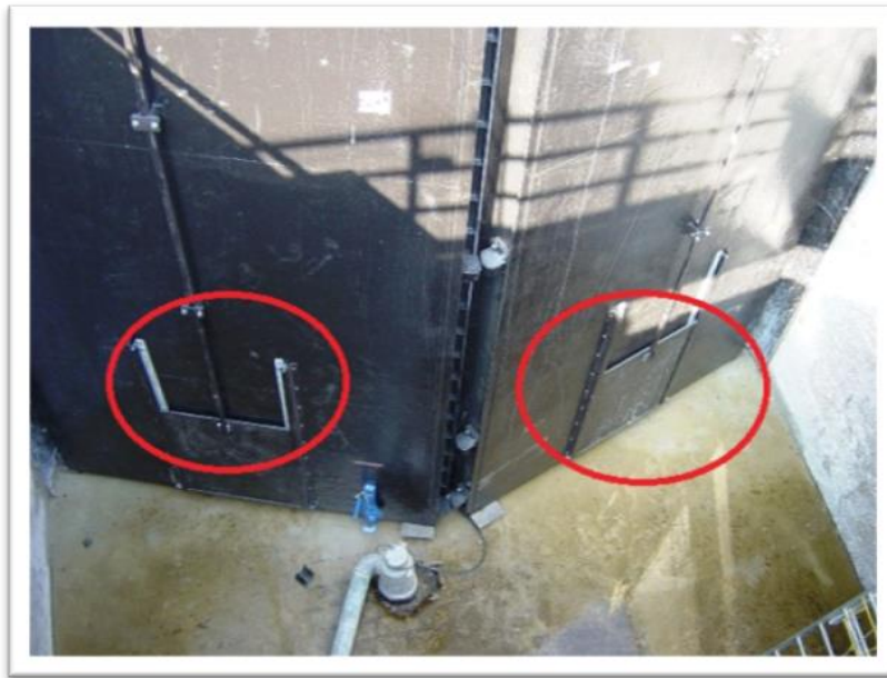
Photo n° 32: Mechanism of the door sluices (doc. Internet)
