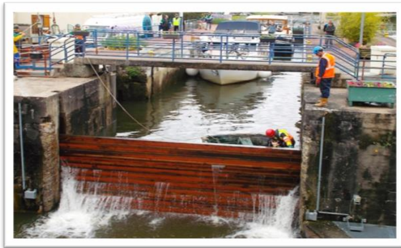
Photo n° 36: Risk related to the setting of a cofferdam (doc. Internet)
