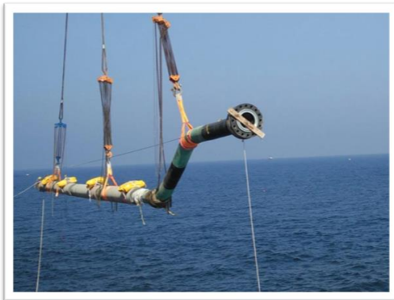
Photo n° 52: Illustration of a correct flange protection (extract photo doc. Terence Elding)
