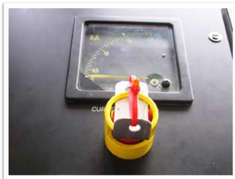
Photo n° 6: Example of an electrical lockout (doc. Internet)
