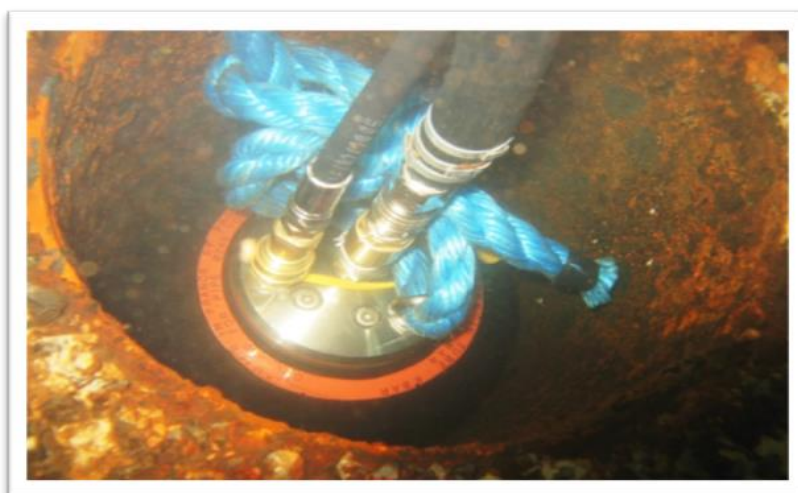
Photo n° 58: Installation of a redundancy plate
