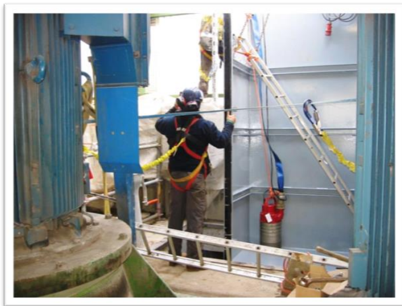
Photo n° 25: Segment valve to be replaced
