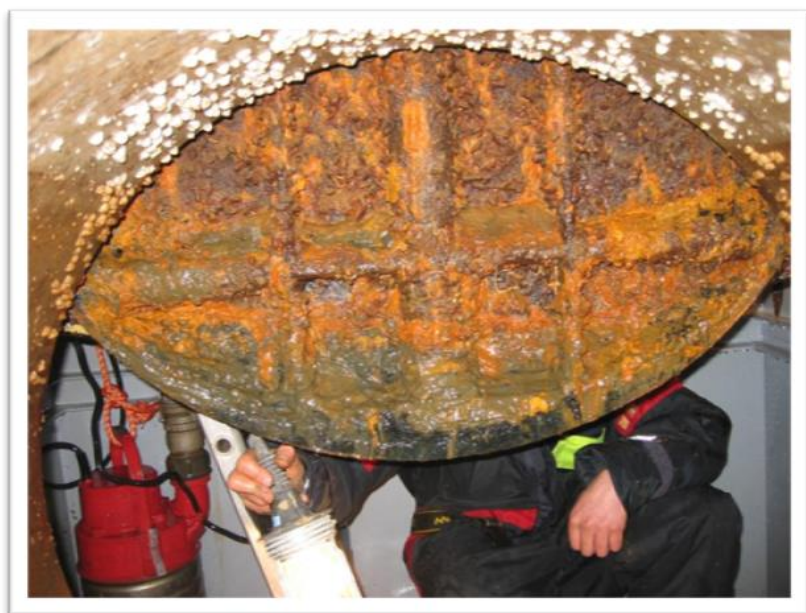
Photo n° 25: Segment valve to be replaced
