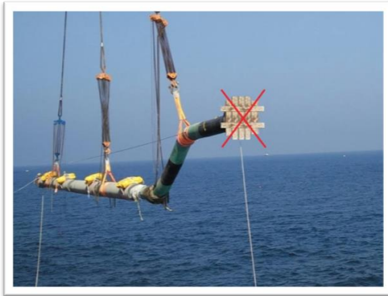
Photo n° 52: Illustration of a correct flange protection (extract photo doc. Terence Elding)
