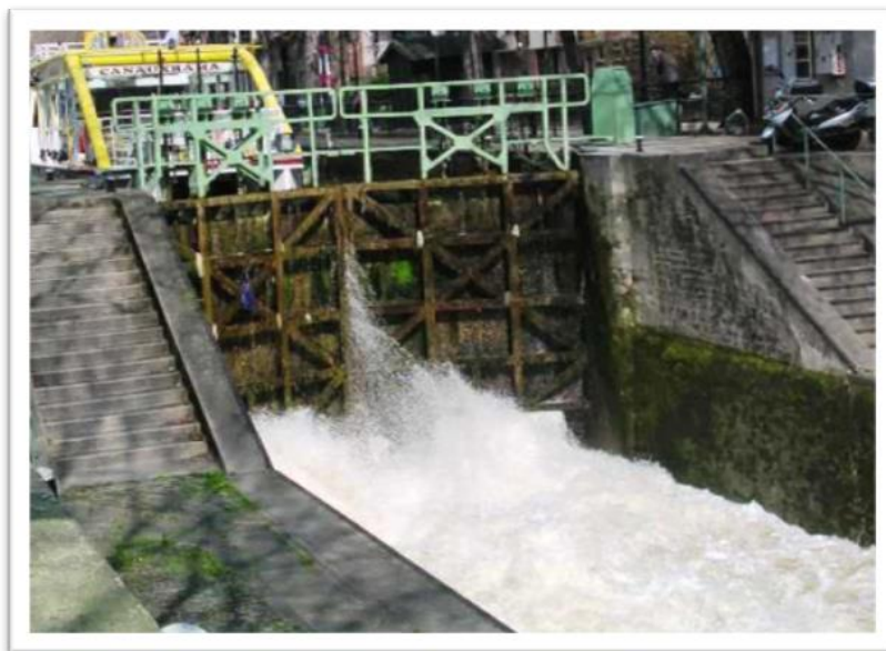
Photo n° 33: Flow through the door sluices (doc. Internet)
