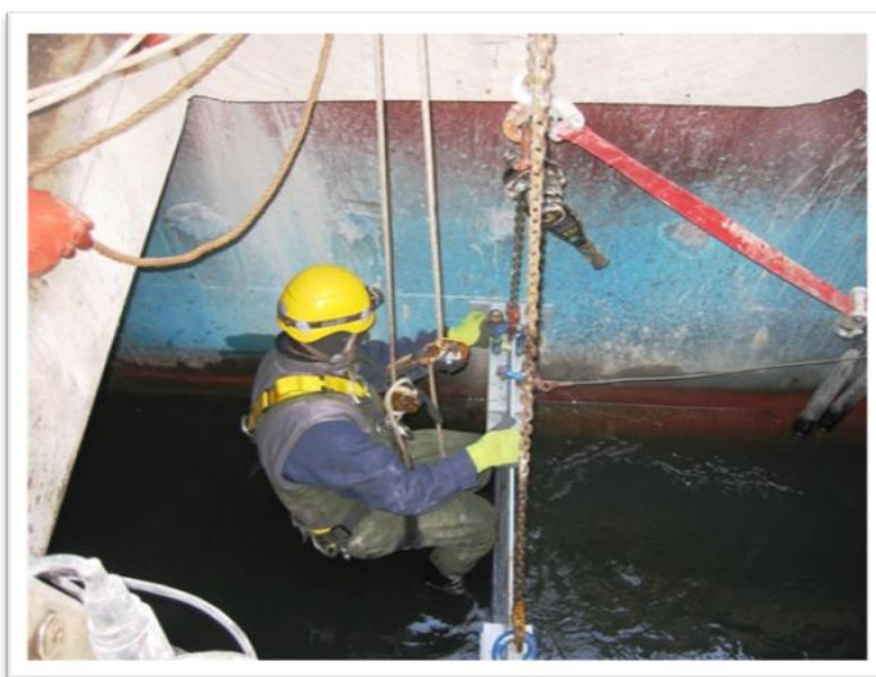
Photo n° 21: Installation of the deflector
