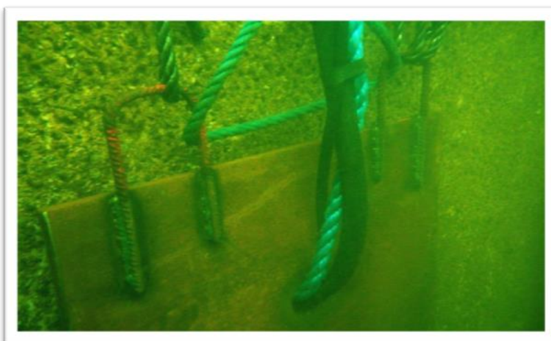
Fig. n°31: Illustration of the installation of a shutter and redundancy plate
