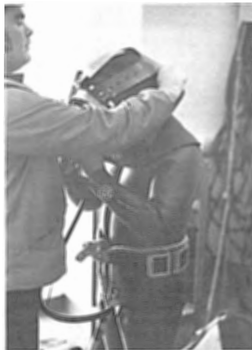
D The diver holds the mask in position while the tender secures the spider.
