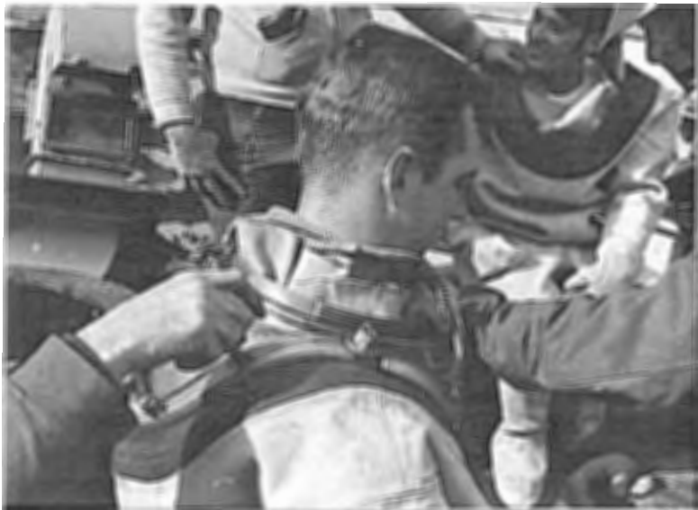
I The four breastplate straps (brales) are placed over the breastplate studs—each in its specific numbered location. Note the hose ties tucked out of the way in back of the diver's neck. The lug nuts are installed hand tight.
