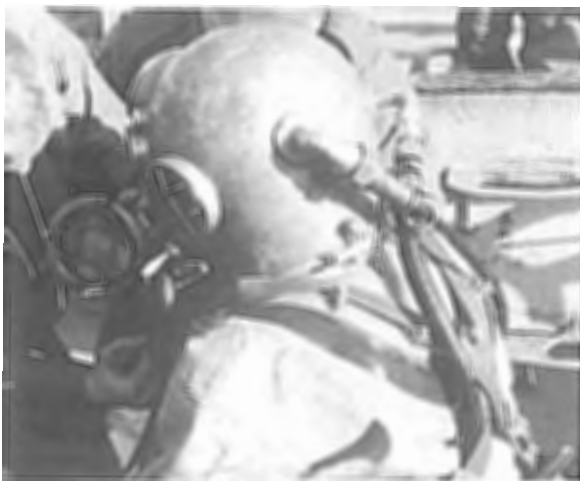
P A tender makes final adjustments. Note hose, lifeline—cable position.
