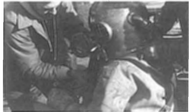
O One tender secures the dumbbell safety lock; the other begins to install the hose group.
